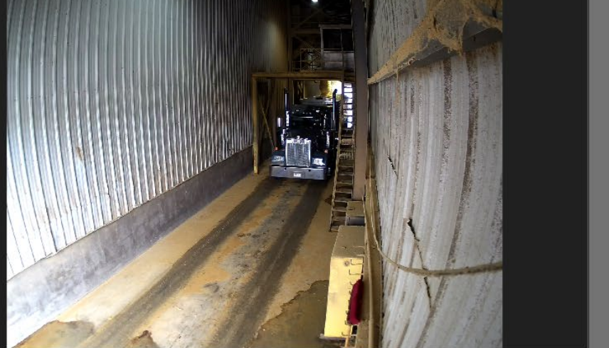
DDG Tunnel 9/28/2023 2:14:17 PM
