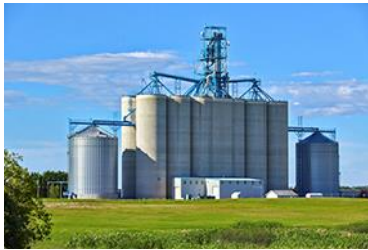
Off-farm commercial grain storage facility.
